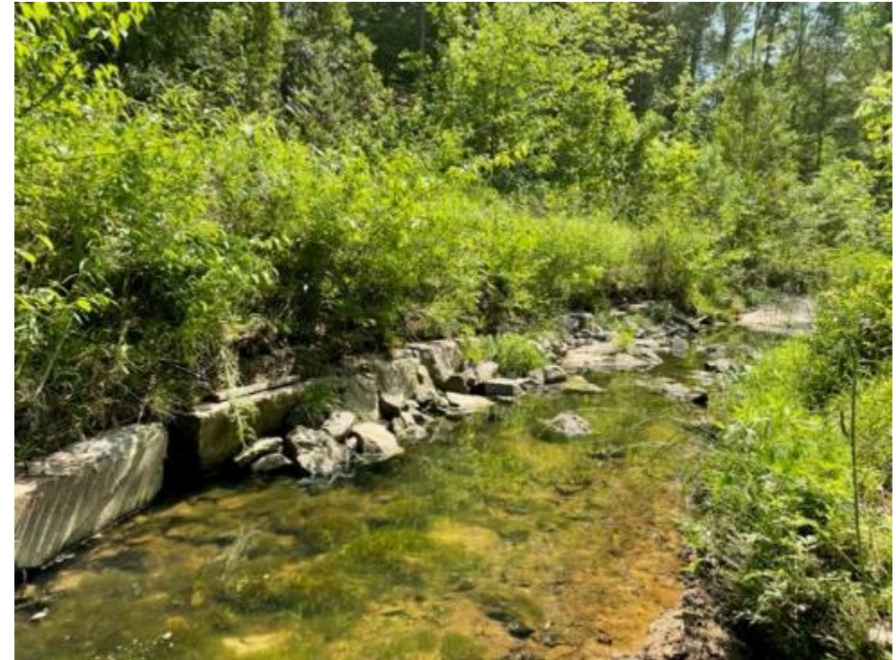
Rock toe with a vegetated Geogrid
