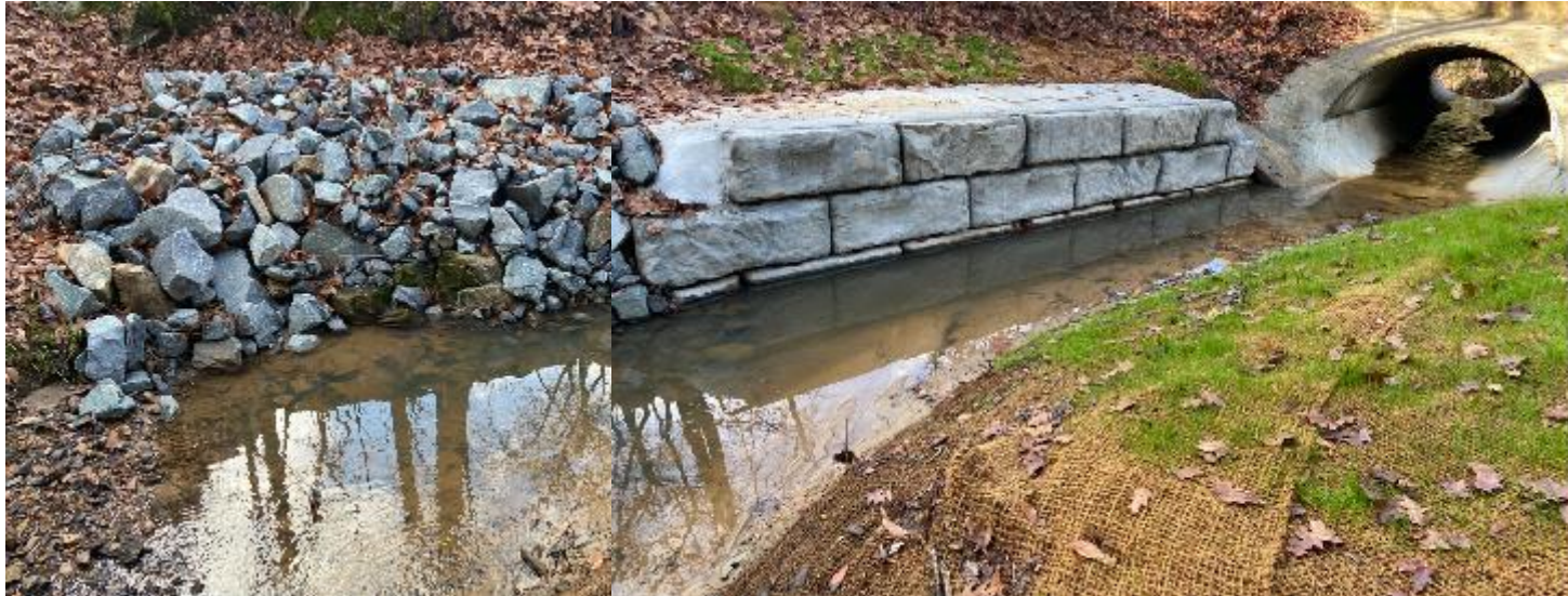
Hard bank Stabilization
