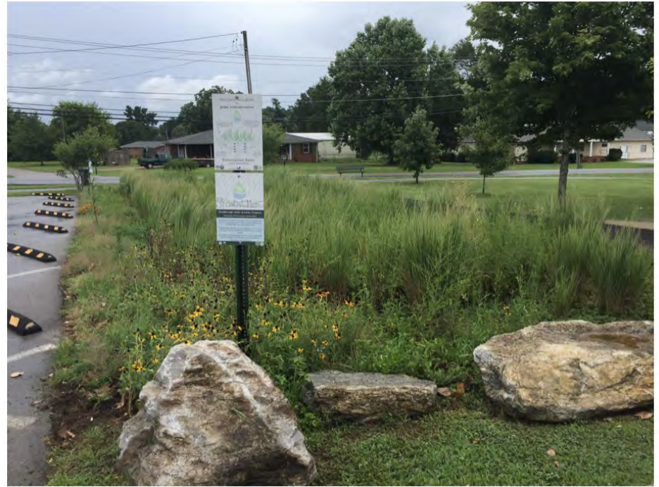
● Bioretention basin at John A. Patten Rec Center
